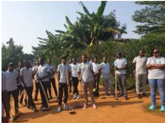
OAG Rwanda Staff getting ready to work on building the connecting roads in the Akagasera Village
